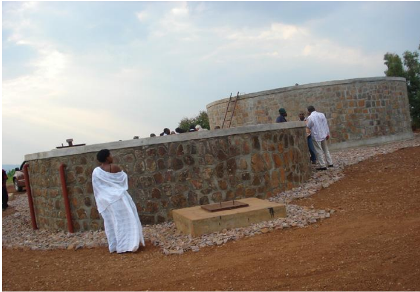
Figure 2: Rubona main water supply tanks constructed through CDF funding
