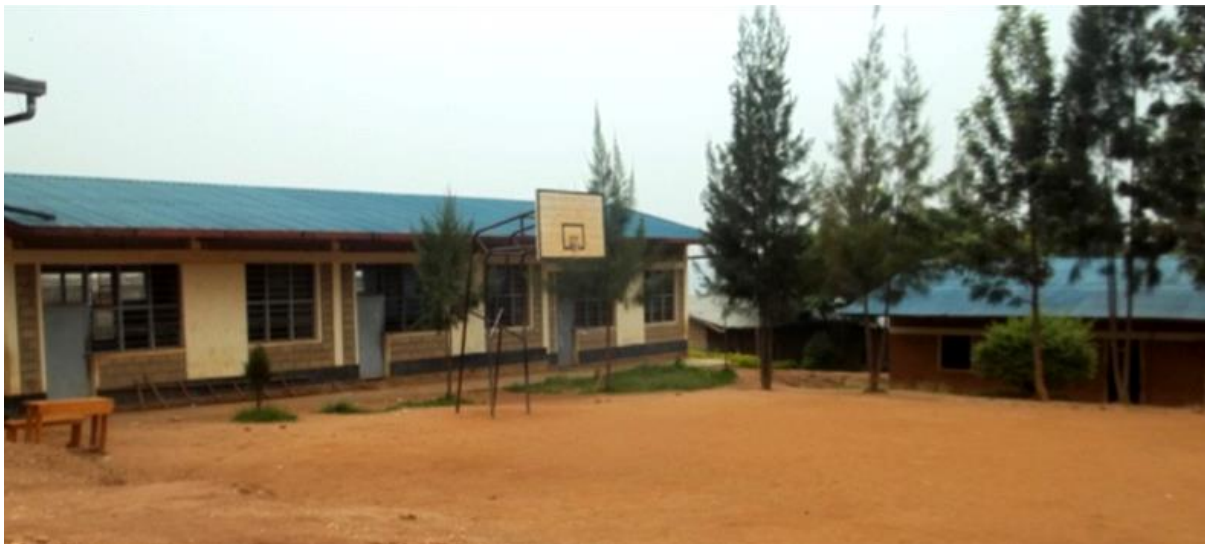
Picture of a school constructed in Remera sector, Gasabo District for 12 Year Basic Education Programme, May 2011
